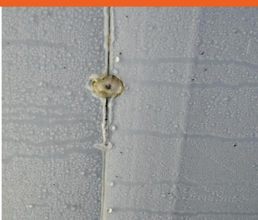
Leaky and unmaintained coolers can become a serious crosscontamination problem. Look out for and control the presence of condensation or drops of water falling from the roof or cooling units or formed on cold room curtains.
